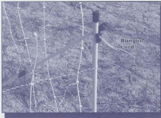
Figure 5—Bungee cords can be used to hold diagonal braces against corner posts.
