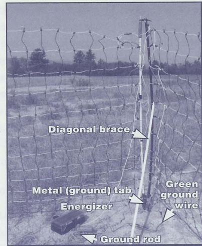
Figure 8—Connect the ends of the fence and attach the energizer to the fence and the ground rod. The ground rod should be at least 1 foot long. If the soil is dry, pour water near the rod to ensure a good electrical ground.
